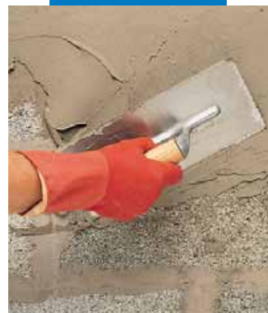
Application of Idrosilex Pronto by trowel
