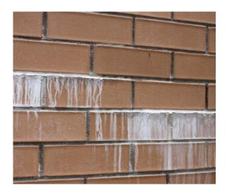
using Efflock in mortar that is compiled with washed sand (without clay) and hydrated lime as a plasticiser. It was found that the accelerant effect can be avoided by substituting lime with clay, but the use of clay should be signed off by a structural engineer and/or tested under the relevant standard (i.e. AS 3700) to confirm satisfactory performance.
