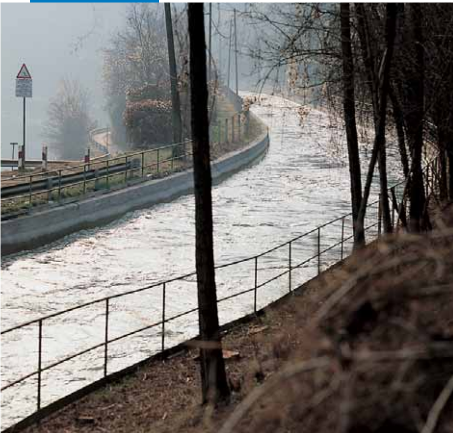
Bertini hydroelectric canal - Como - Italy. Surfaces treated with Idrosilex Pronto
