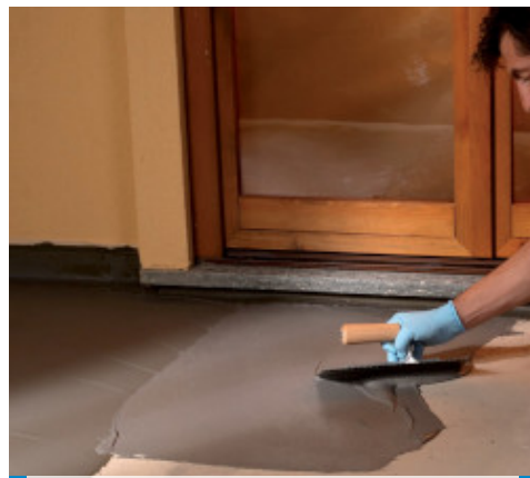
Waterproofing of terraces by trowel
