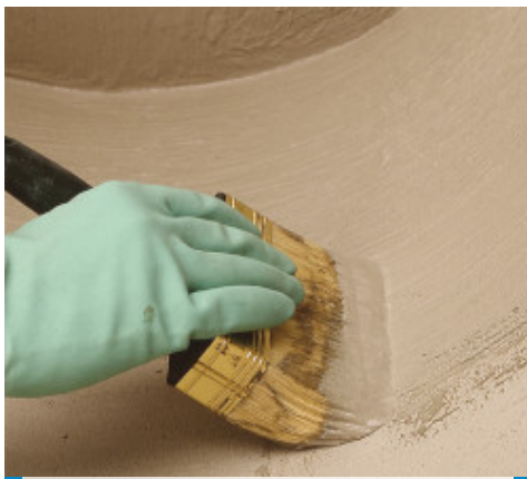
Waterproofing of details by brush
