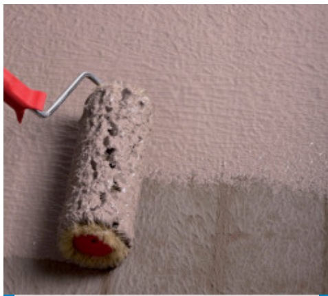
Waterproofing of details by roller
