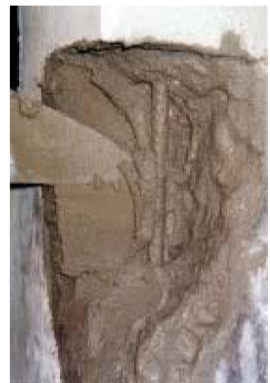
Apply the mortar
