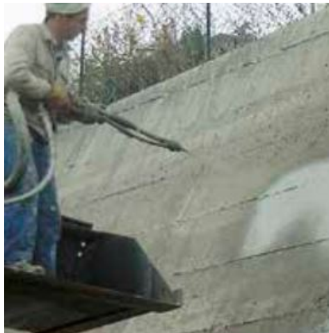
Application of Planiseal 88 by spray gun in hydroelectric canal
