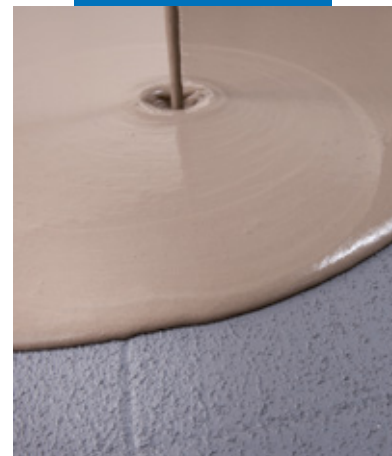
Application of Ultraplan self-levelling smoothing compound on dry Eco Prim Grip on old floor
